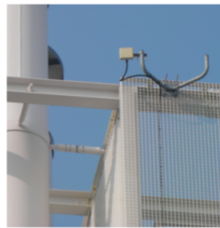
Fig. 3. Installation of antenna at Future University Hakodate (FUN).
