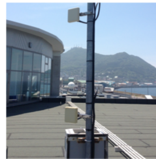
Fig. 4. Installation of antenna at Hakodate Research Center for Fisheries and Oceans (HRCFO).
