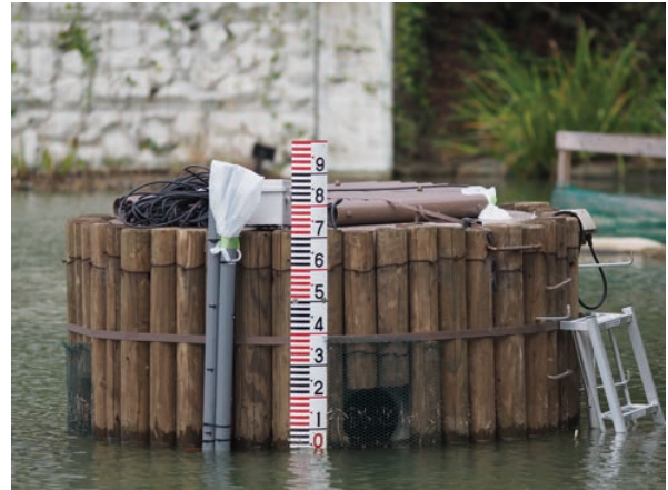
Figure 7. installed eTape, pressure gage and sensor node
