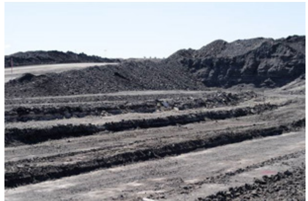
Fig 6. Photo of multi-tier configuration excavated for the GPR evaluation.
