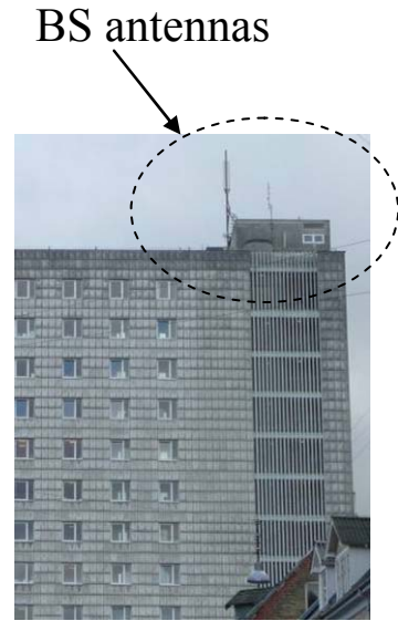
Figure 4: Base station on the building
