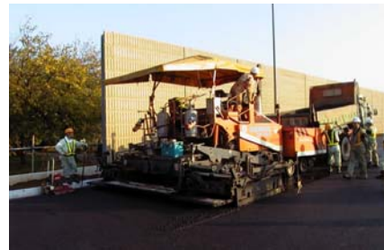
Figure_8 Pavement Condition (Spreading and Levelling)
