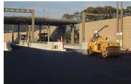
Figure_9 Pavement Condition (Rolling)
