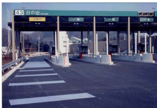
Figure 1 Kenodo Hinode IC, ETC Toll Booth (September, 2001, Actualization of the Electromagnetic Wave Absorbing Pavement)
