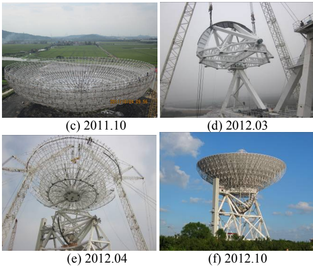
Figure 5 Assembly of the SHAO 65m radio telescope antenna.
