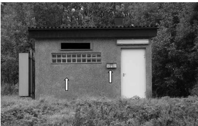
Fig. 3 An older generation of control facility (hereby called CF1). Some important points have been marked.
