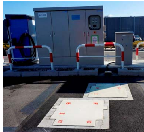
Fig. 2 Prototype of the transmitting circuits and pads
