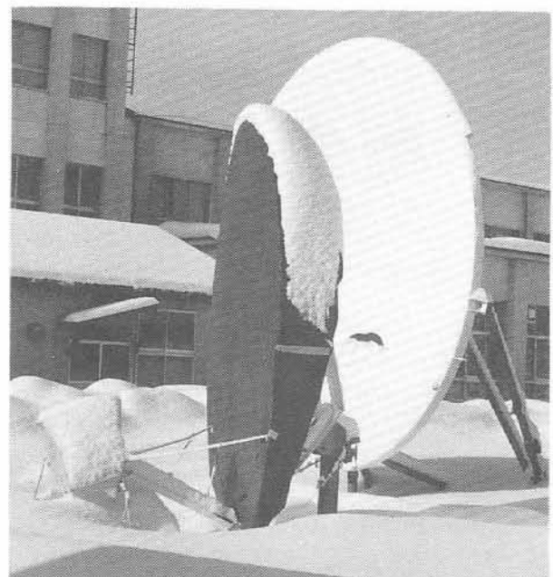
Fig.6 Example of 1.8m diameter NGS off-set type antenna.
