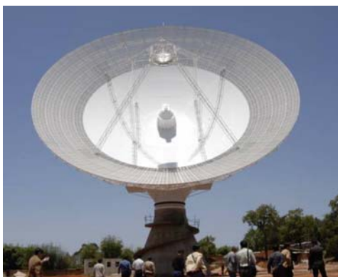
Figure 3. Picture of the 40m reflector antenna
