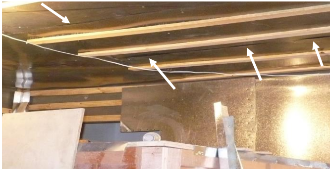
Fig. 1. Shielding with bad connections between plates joints, creating unwanted gaps (white arrows).
