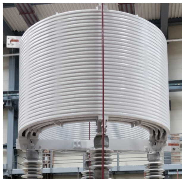
Fig. 1 Photograph of actual air core reactor.
