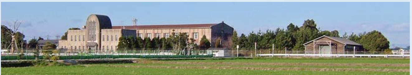
Yosami Radio Transmitting Station
