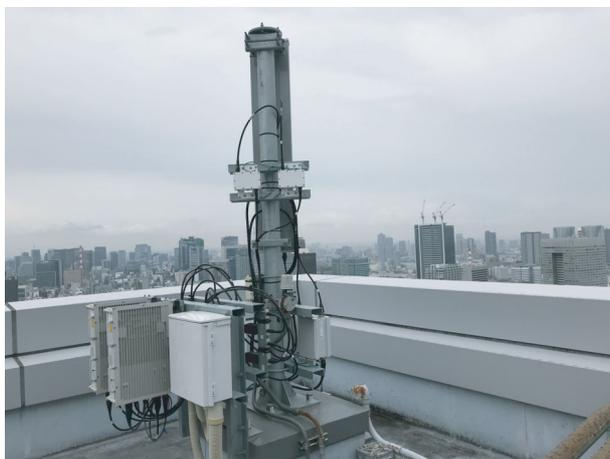
Figure 3 Appearance of the Wide-area Station The BBU and routers are installed inside the building.
