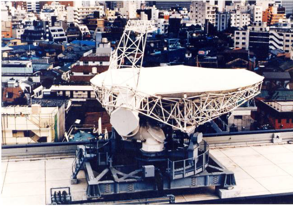
Figure 3: Commercial offset Cassegrain antenna with 11.5m diameter on the roof top of Shinjyuku regional center.
