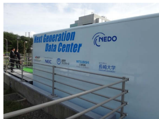
Fig. 1 Next generation module type data center.
