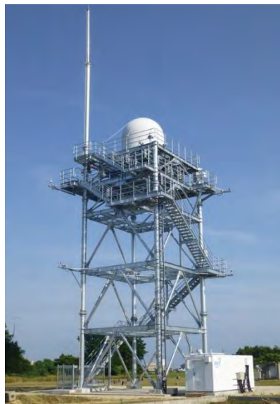
Fig. 7 Phased Array Weather Radar installed in Kobe city
