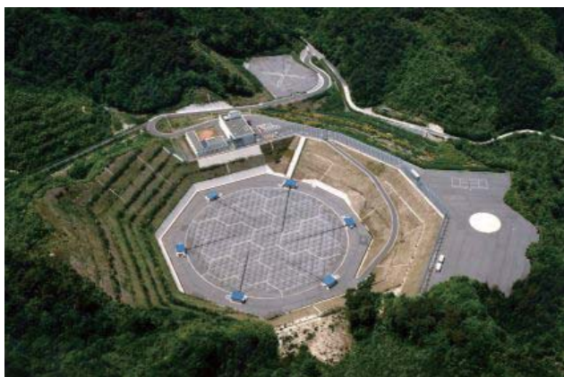
Fig. 1 Overview of the MU radar. The circle with a diameter of 103 m is the antenna array
