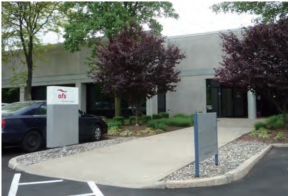
Fig. 1 Building of OFS Laboratories
