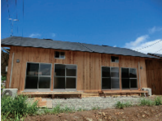
Fig. 2 Temporary housing unit in Iwaki-City.
