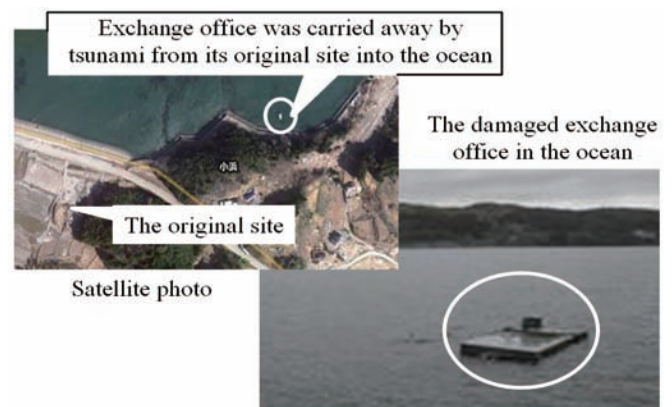
Fig. 2 The Damaged Tokura Exchange Office, in Miyagi Pref.
