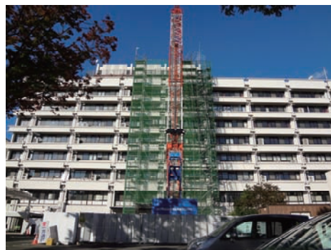
Fig. 1 No.1 faculty building waiting for demolition.
