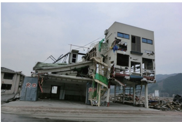
Fig. 4 Otsuchi Fire Station (Flooding depth is estimated at 10 meters or higher.)
