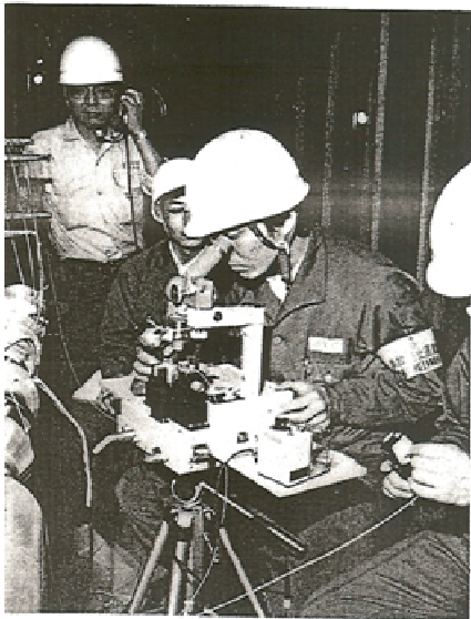
Fig. 6 Construction of optical cable route (FR1 1978)
