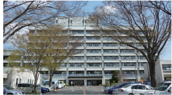
Fig. 1 Damaged No.1 faculty building.
